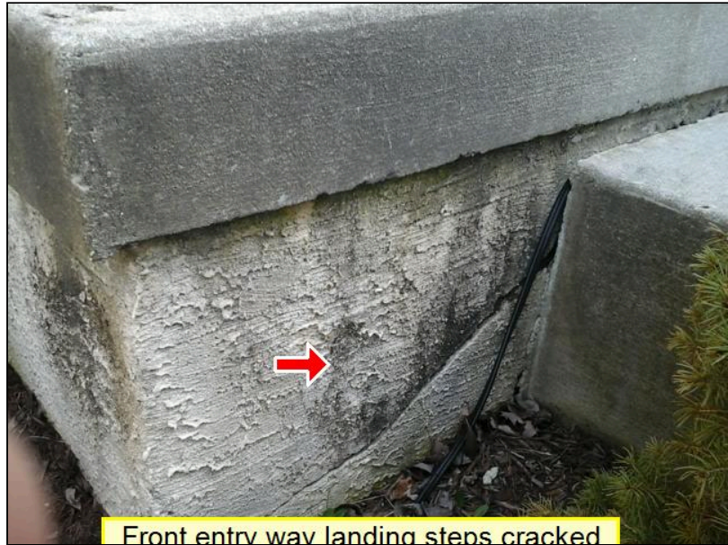
2.3 Item 2(Picture) Cracked Foundation
