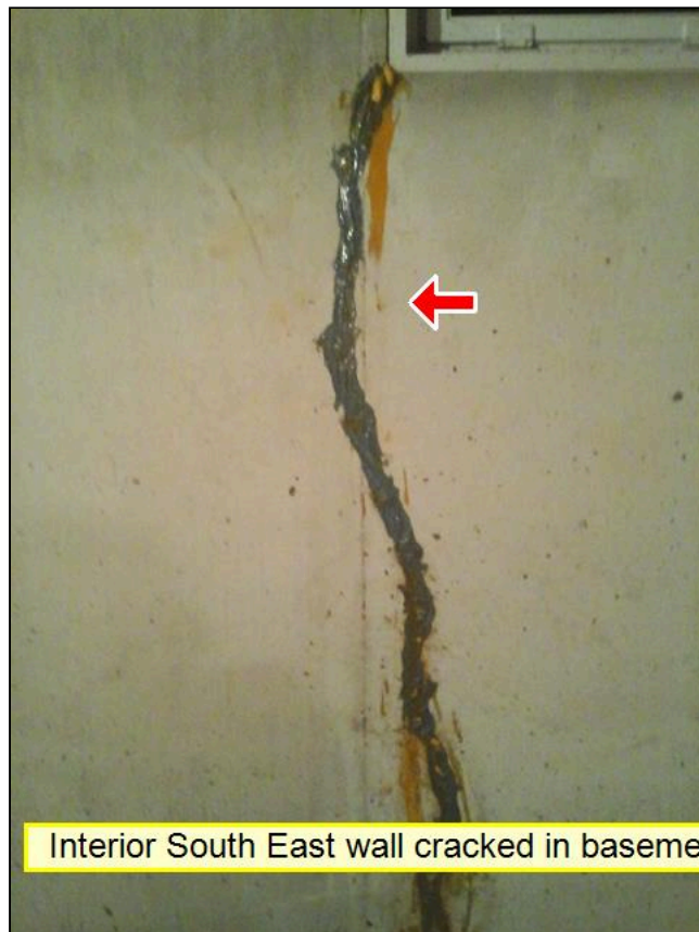
7.0 Item 2(Picture) Basement Wall Crack
