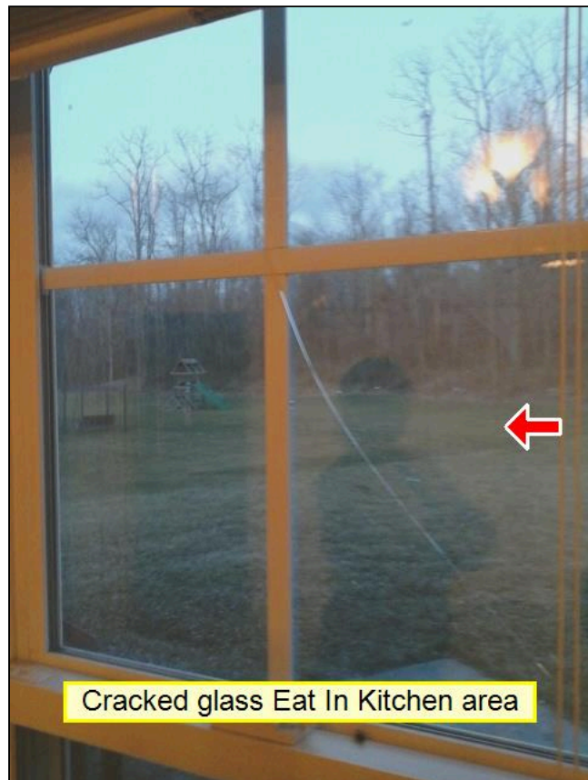
6.2 Item 1(Picture) Cracked glass in Kitchen
