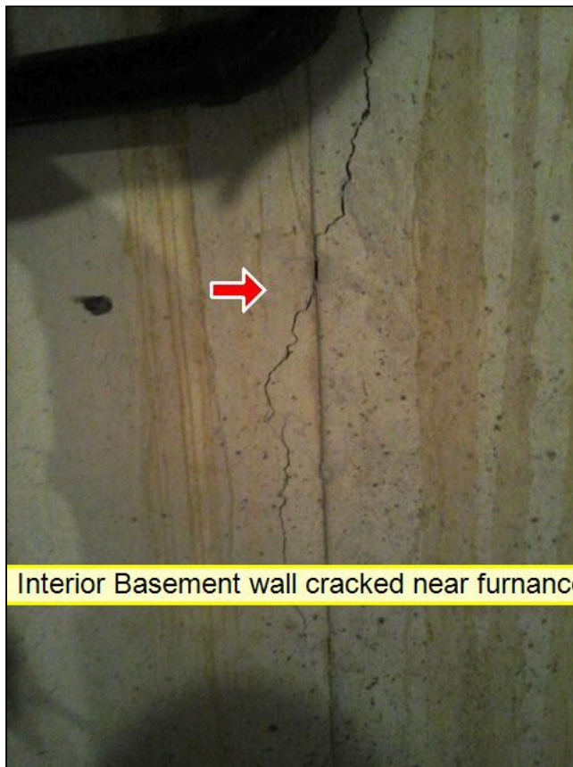
7.0 Item 3(Picture) Basement Wall crack
