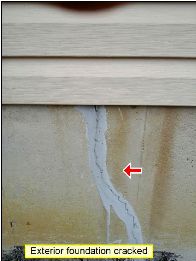
7.0 Item 1(Picture) Basement wall crack
