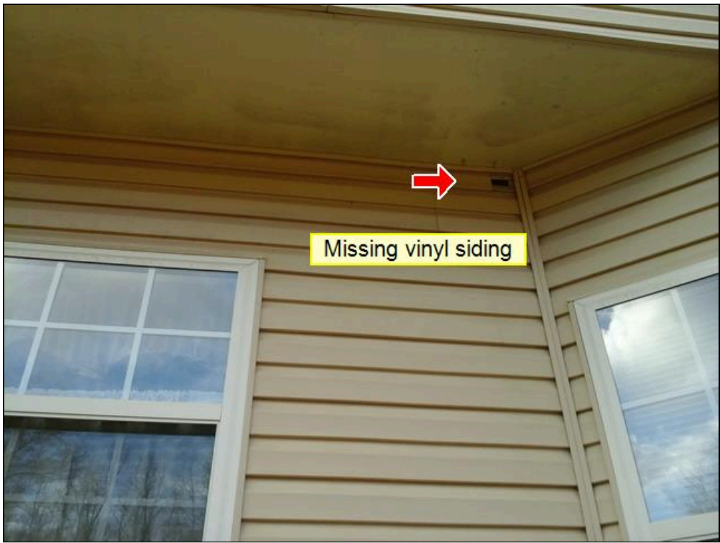
2.0 Item 1(Picture) Missing siding
