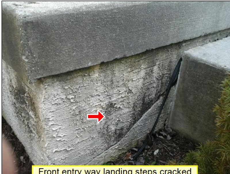
Front entry way landing steps cracked
