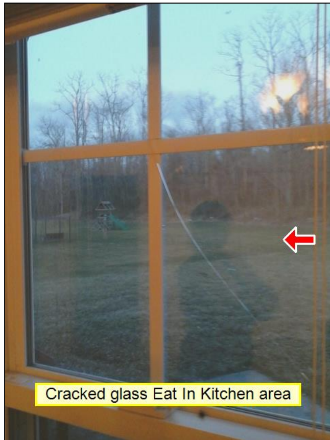
6.2 Item 1(Picture) Cracked glass in Kitchen
