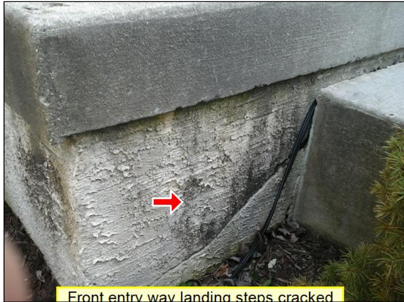
Front entry way landing steps cracked
