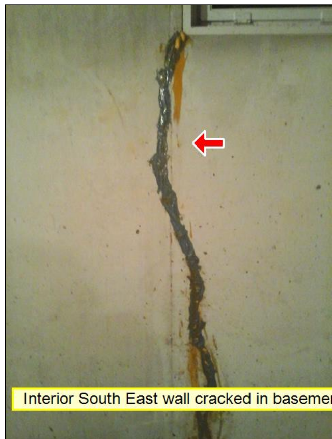
7.0 Item 2(Picture) Basement Wall Crack
