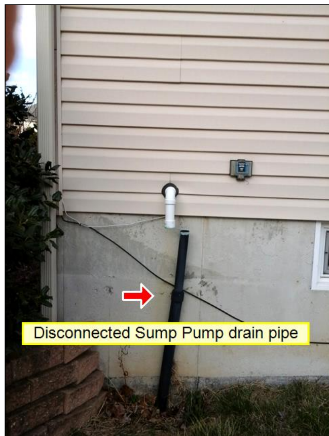
8.6 Item 1(Picture) Sump pump drain
