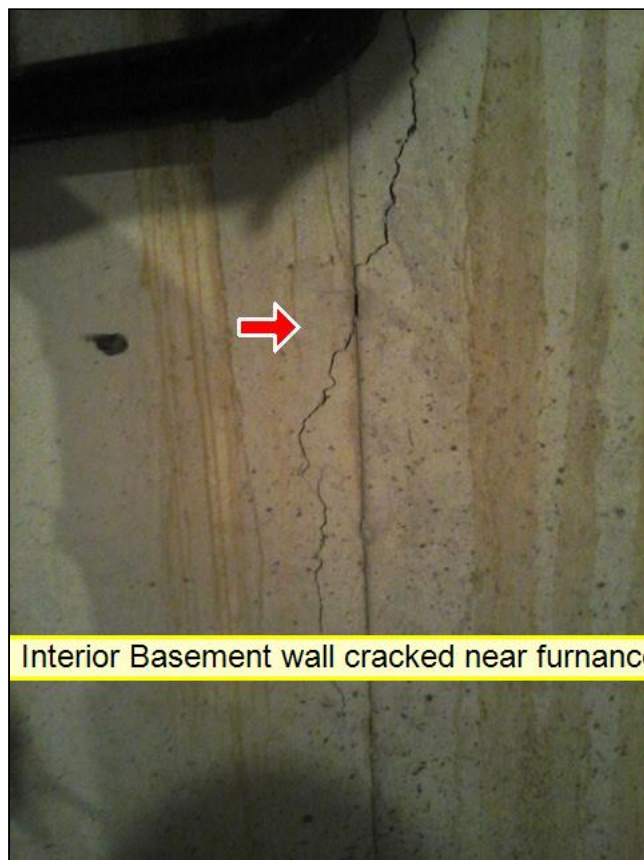
7.0 Item 3(Picture) Basement Wall crack
