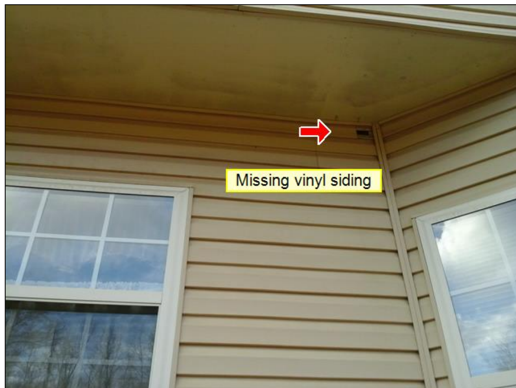
2.0 Item 1(Picture) Missing siding
