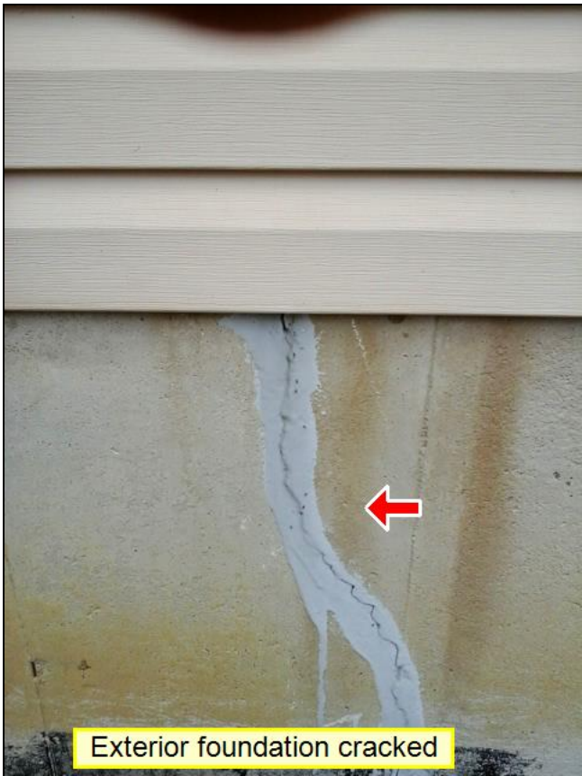
7.0 Item 1(Picture) Basement wall crack
