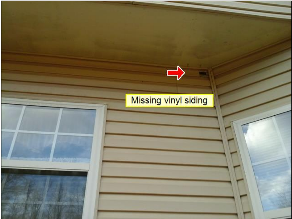
2.0 Item 1(Picture) Missing siding
