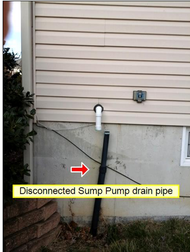
8.6 Item 1(Picture) Sump pump drain
