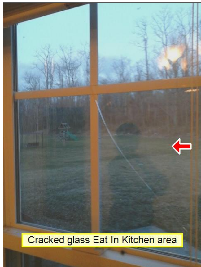
6.2 Item 1(Picture) Cracked glass in Kitchen
