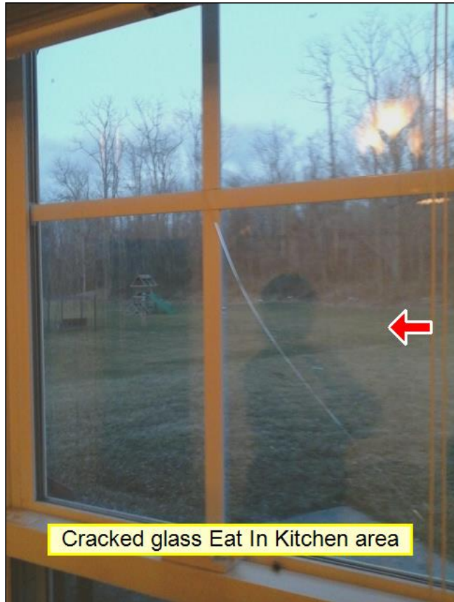
6.2 Item 1(Picture) Cracked glass in Kitchen
